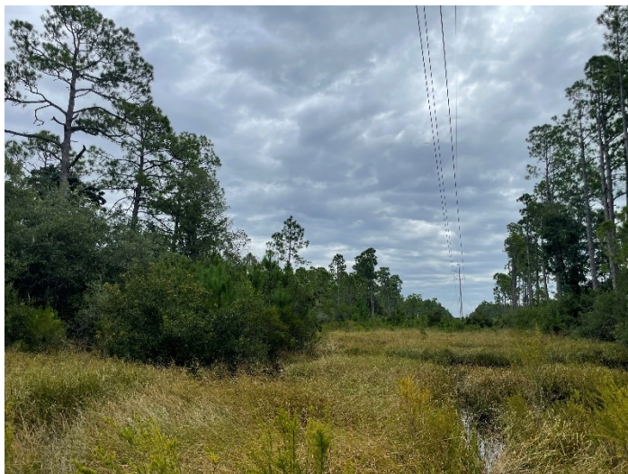
Powerline Easement (Typical) – September 2024
